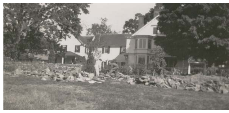
Construction of the Formal Garden wall, c. 1915.
